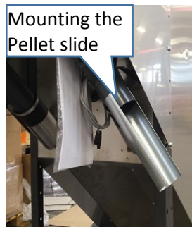
Installation temporary pellet storage, connecting the Maulwurf, mounting the Pelletslide. Fig 14
